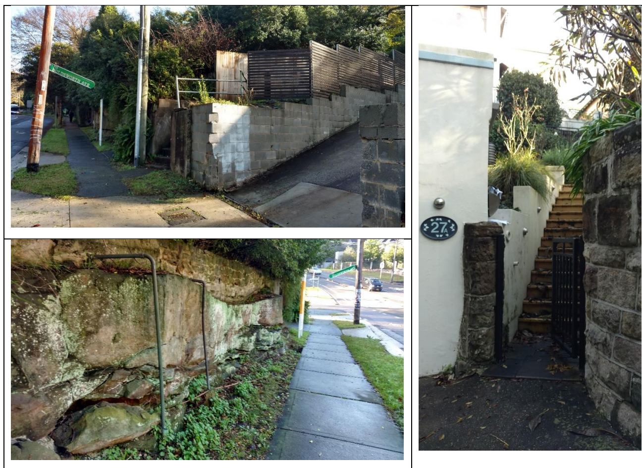
Figure 1: Stage 1 Site photographs (southern portions and 27 Holdsworth Avenue (right))
